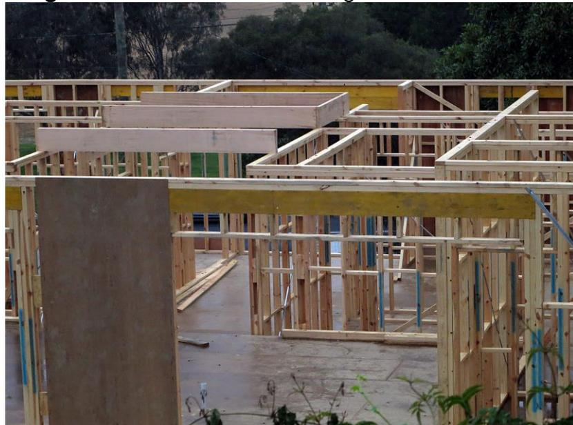
**Image:** Timber house structure using F17 Mountain Ash and Pine timbers.
